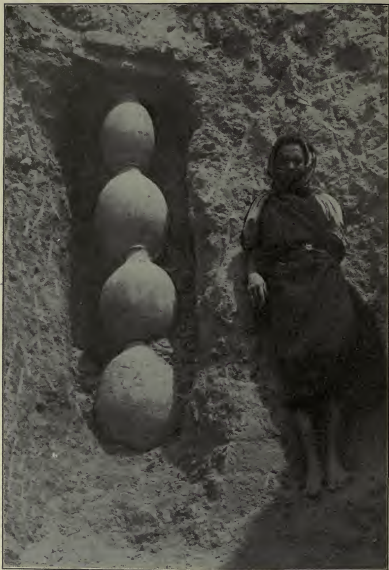
Perpendicular Drain composed of Jars. About 200 B. C.
